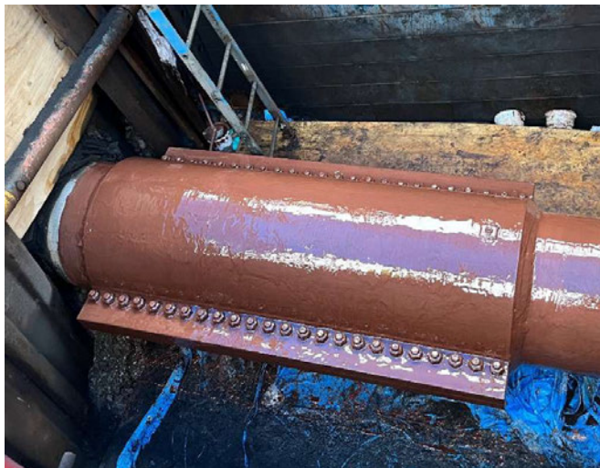
Figure 2: Pipeline excavation in [REDACTED]
