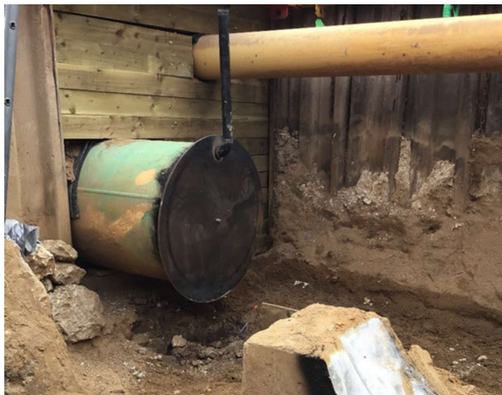
Figure 3: Pipeline excavation at [REDACTED] gas compressor station.
